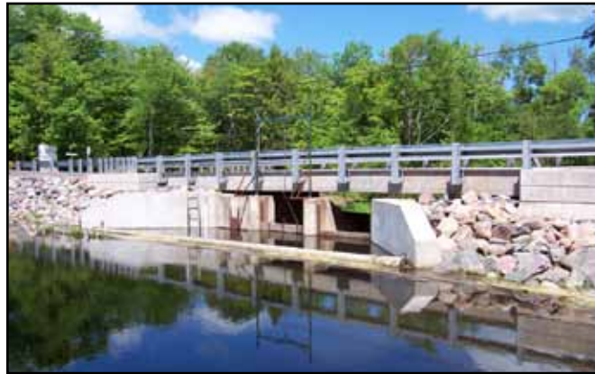
Intake of Water flowing into Cisco Dam
