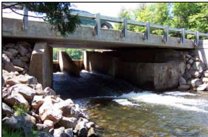
Outtake of Water Flowing from Cisco Dam
